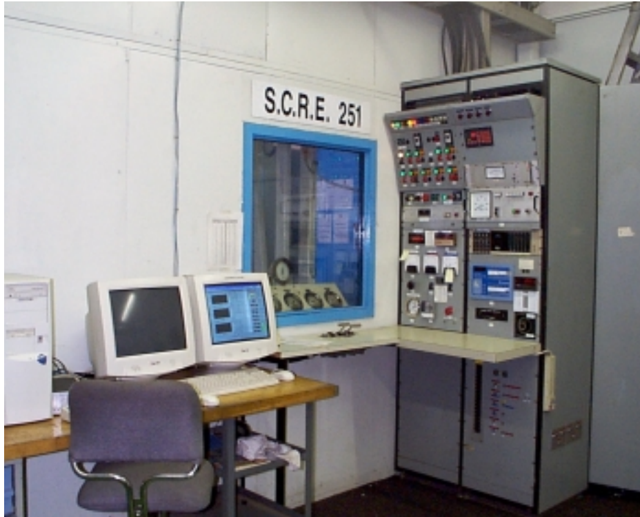
C-2: Control Unit
